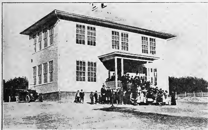
A HAPPY COMMUNITY CENTER IN OLD POWELL FORT, SHENANDOAH COUNTY
